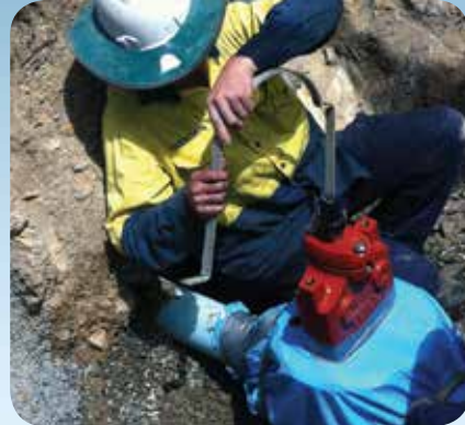
An InsertValve installation under full line pressure.
