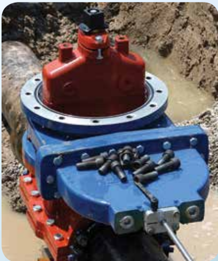
Low-profile bonnet used as line stop.
